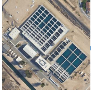
Surface Water Improv. Dist. 4 Water Treatment Plant
